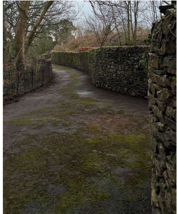
After – Ivy cleared for better 3D laser survey of stone wall
