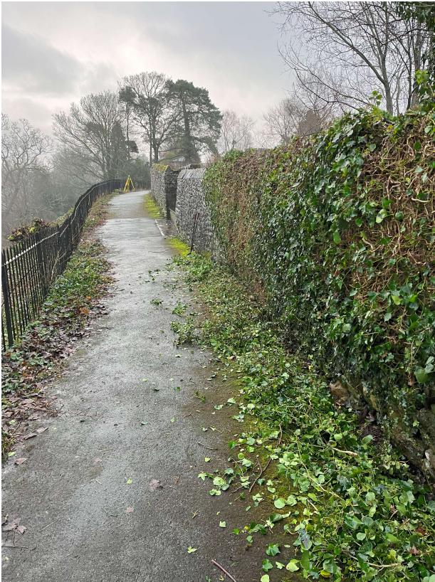
Before – intrusive ivy on the stone retaining wall
